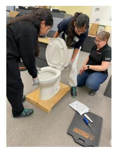
• **Plumbing Workshop:** Students learned the fundamentals of assembling a toilet and installing a faucet by attaching water lines and assembling drainage fittings on a bathroom vanity.
